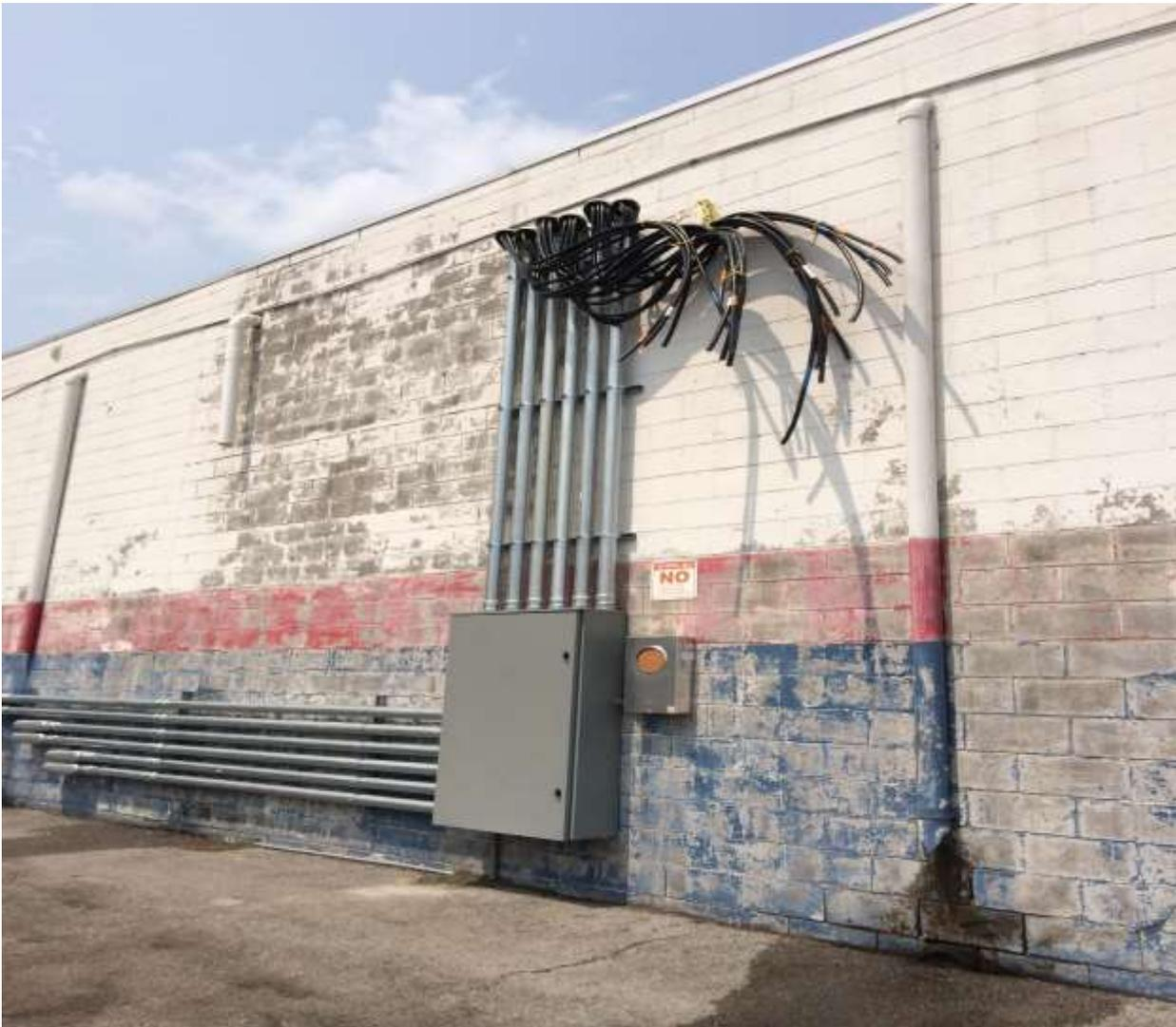
In this scenario, customer has provided ample length for EPB to connect the service, along with clearly marking the phases. Meter center was mounted to where the center of the meter face will be within 4-6 feet above the final grade.
