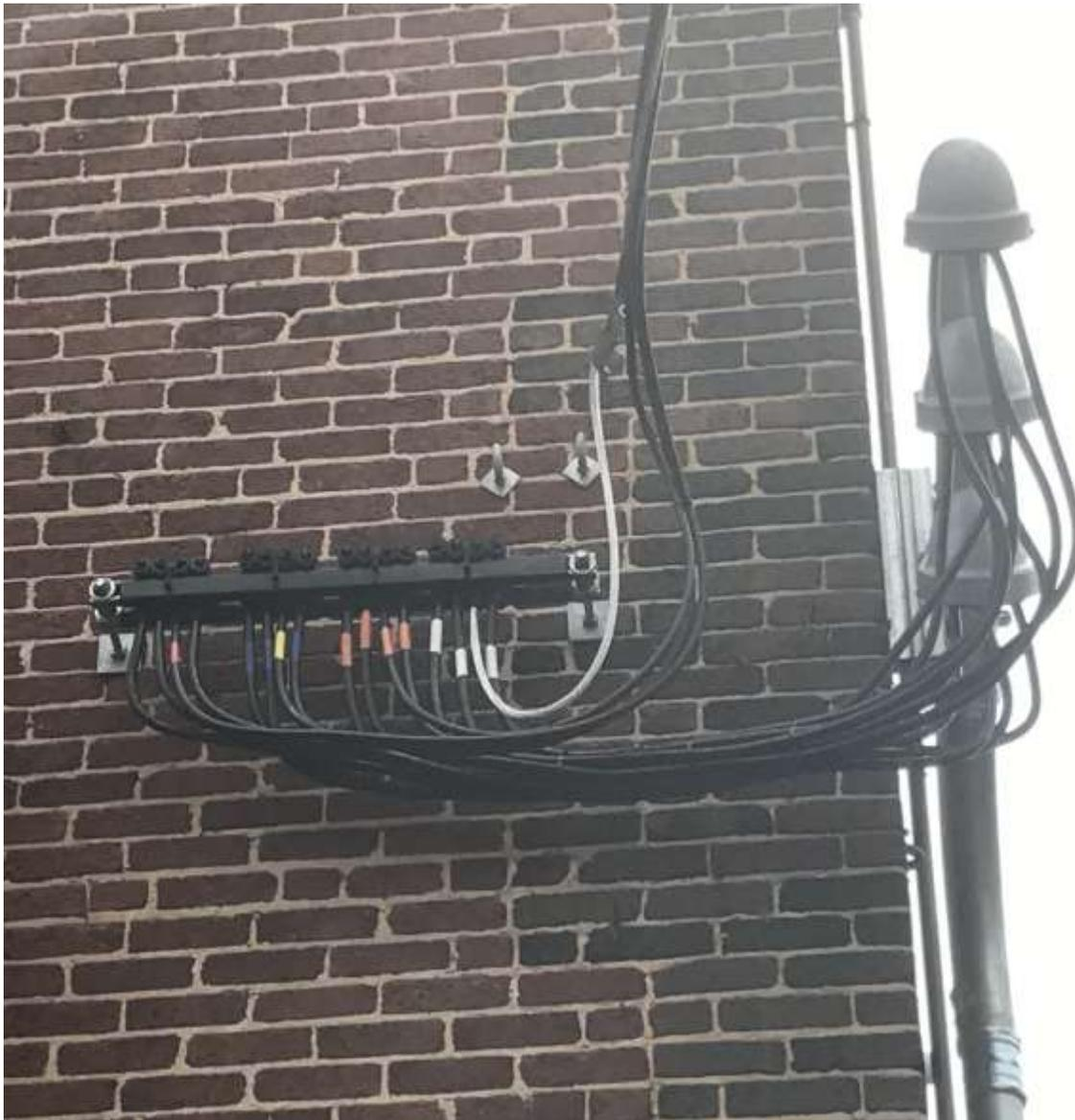
For overhead services containing multiple conductors per phase, EPB will supply a mounting bracket for the PED connectors as seen above. The customer is responsible for mounting the bracket, leaving sufficient length at the weather head, and correctly marking the load side phasing.
